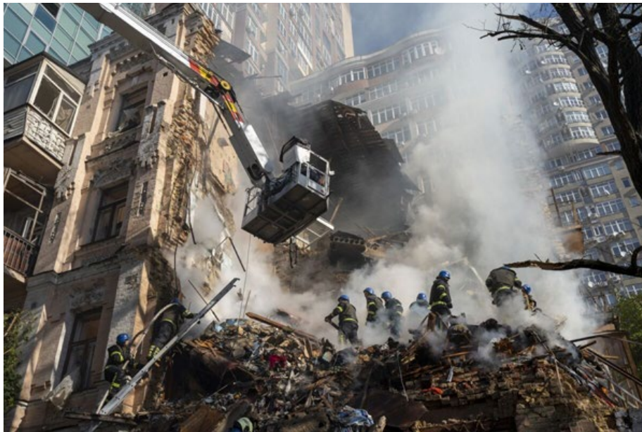
Figure 1. Damage to civilian infrastructure in Ukraine due to Russian Drones
